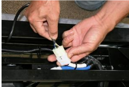
Image 14 – connecting power cord to control box harness
